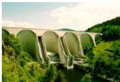
Figure 7: Barrage de Grandval
